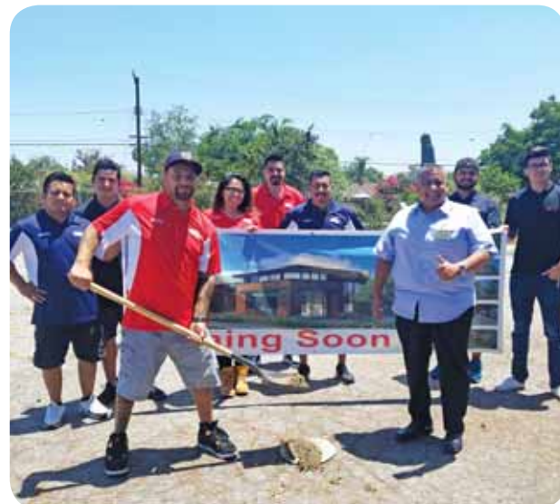
Chamber Board President congratulates Xtreme Tint owner Erick Ramirez and his staff on the ground breaking of their new building which will be located right next door to their existing shop
